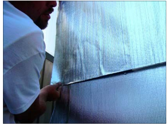
Position FlexClad into place.
