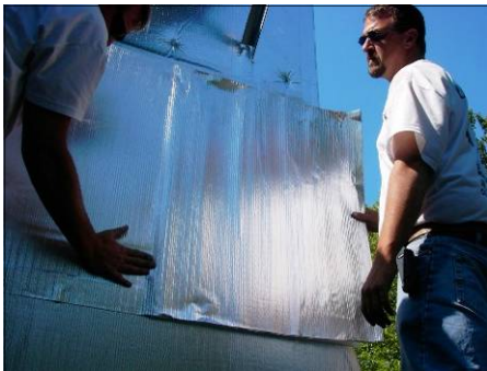
Remove release paper, align membrane and press to stick.
